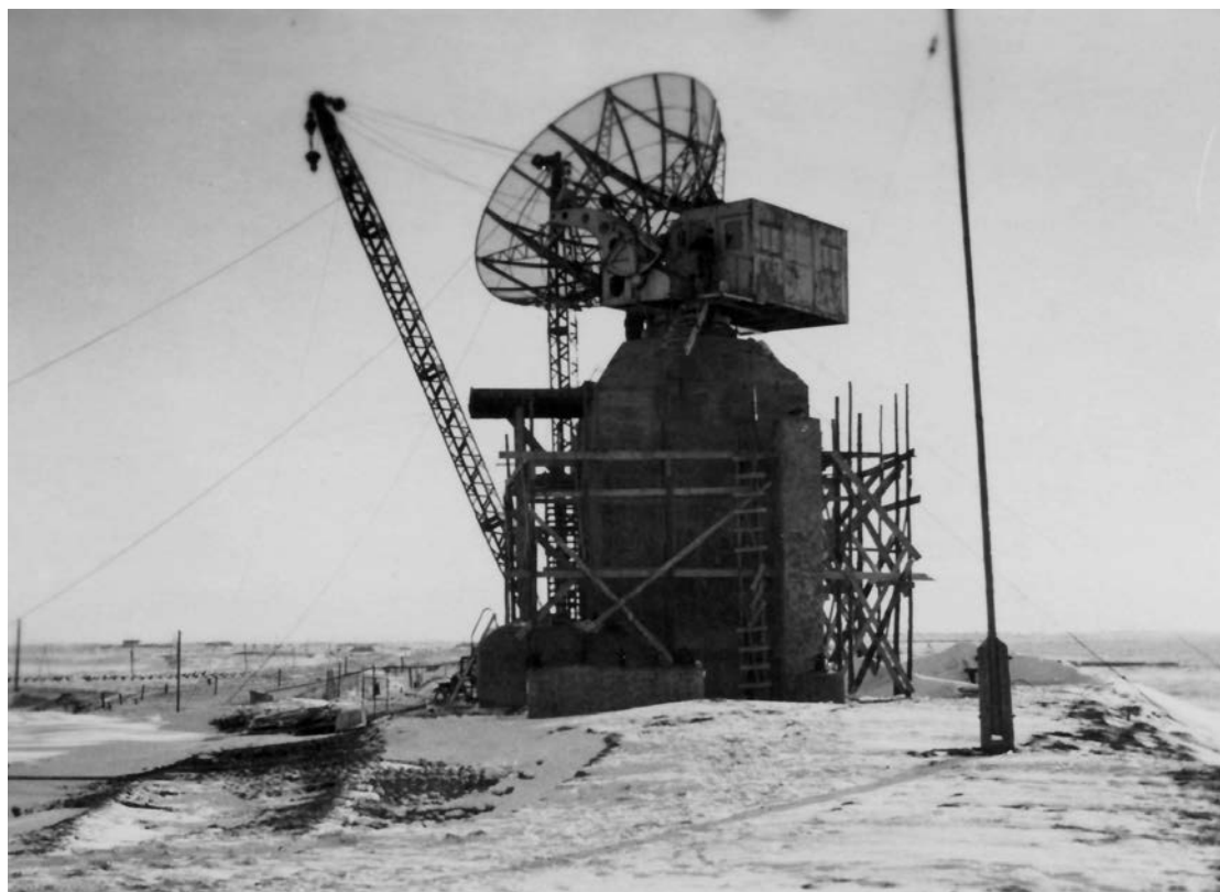
Radar under montering i 1944.
